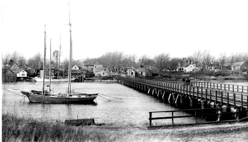
First Bass River Bridge
