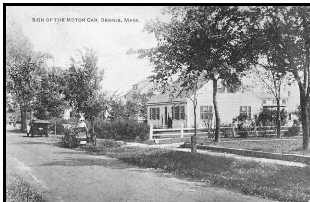
Along Route 6A – The Old King's Highway
