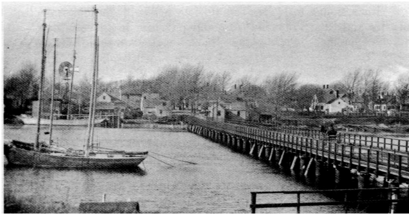
Bass River Bridge
